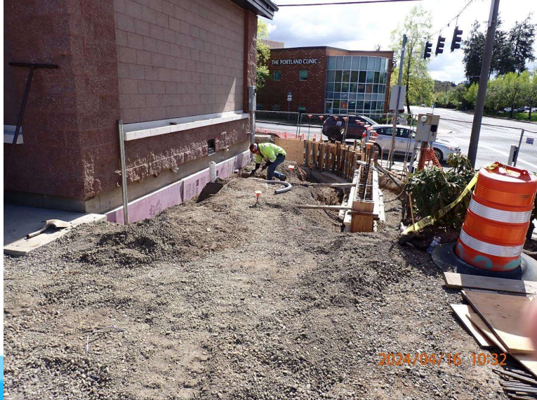
Sitework at exterior of PFC Facility
