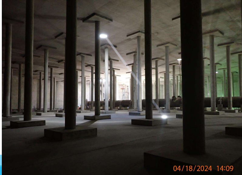
Interior of reservoir tank
