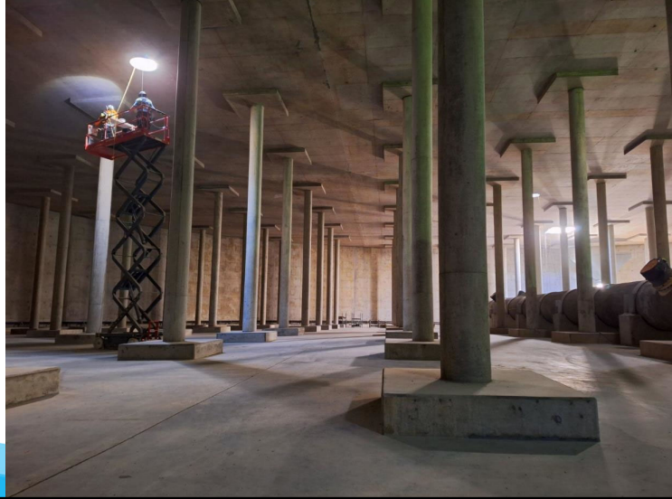
Reservoir tank ceiling touch-up work
