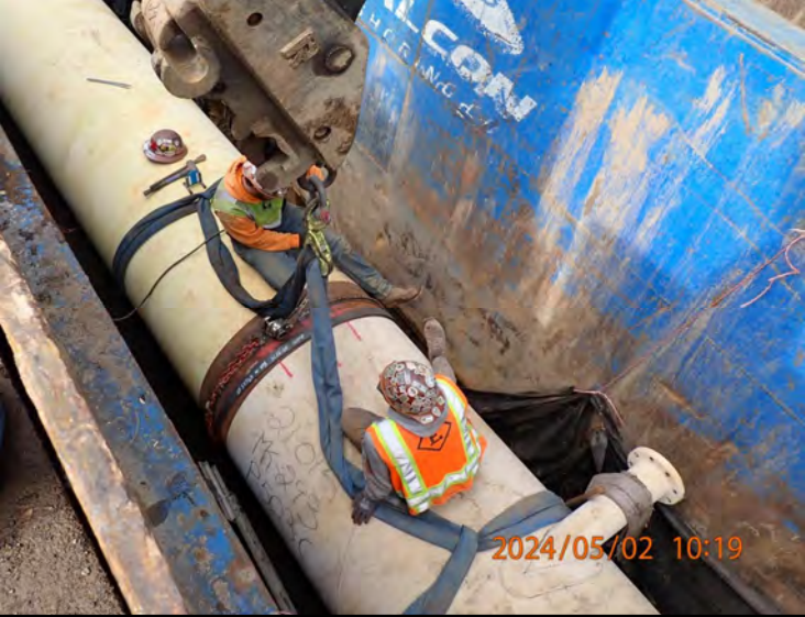
Final section of 48" waterline on Scholls Ferry Rd. near Denney Rd.
