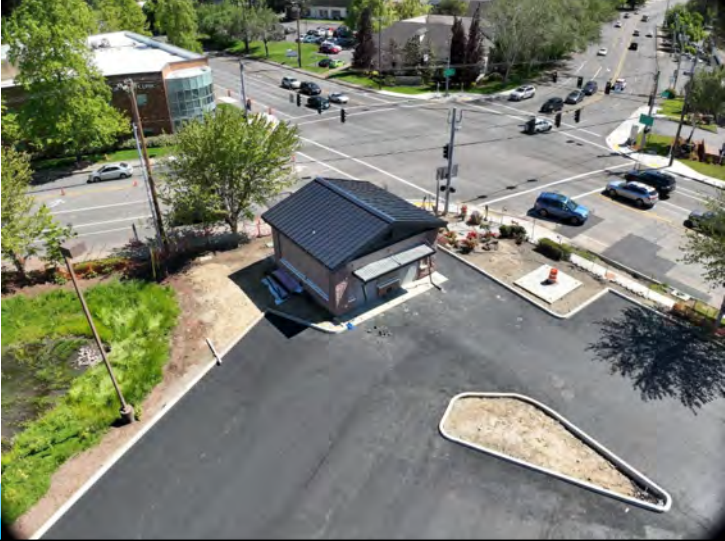
PFC facility – parking lot paved
