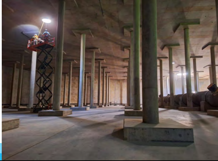
Reservoir tank ceiling touch-up work
