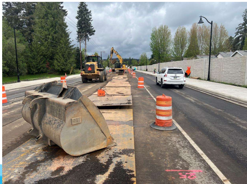
Clean Water Services sewer force main construction
