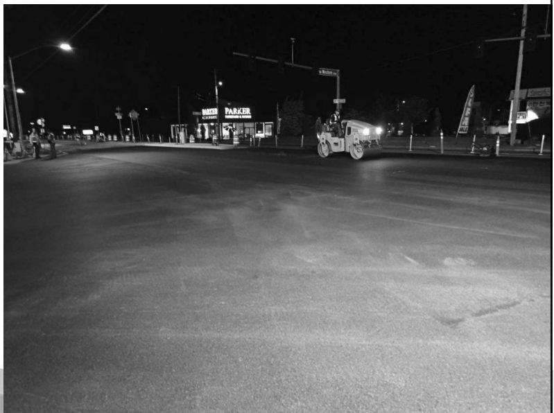
Final paving of Western Avenue / Beaverton-Hillsdale Highway intersection
