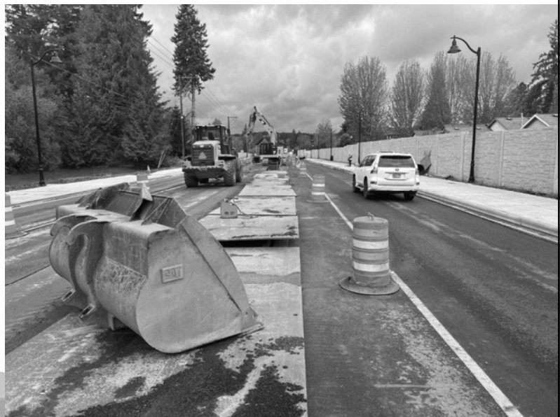
Clean Water Services sewer force main construction
