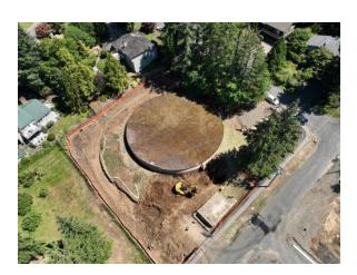
Roof Removal: The reservoir's roof and 40 columns were systematically removed using an excavator equipped with hydraulic shears.
