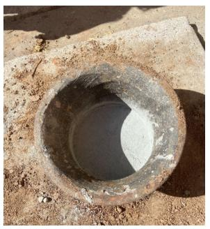
• Safety Measures: Pipes were capped to prevent contamination of the water system and erosion due to groundwater movement.
