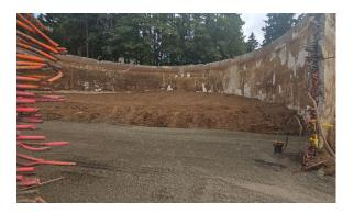
Support Measures: Soil and gravel were backfilled inside the reservoir to support the walls during further demolition.
