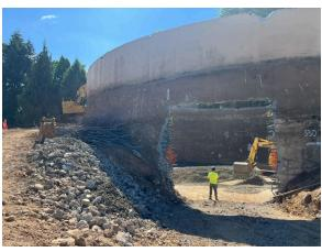
Cleanup Facilitation: A large window was cut into the reservoir's side to remove the roof and column rubble.
