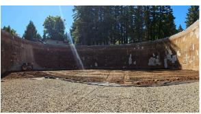
Reservoir Floor: Drain rock and fabric were placed to manage water drainage and stabilize the floor.
