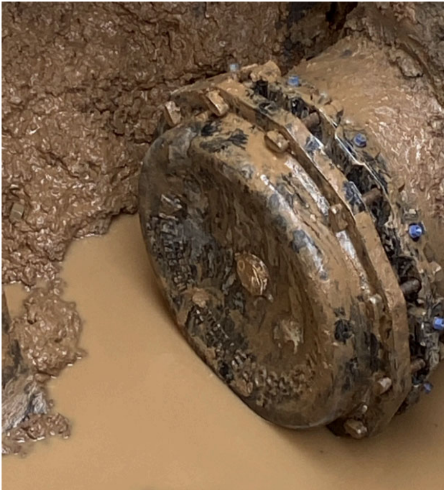
Capped the water main leading to the existing reservoir.
