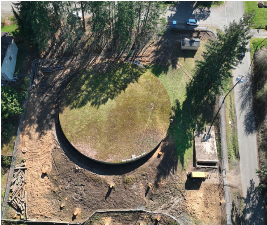
Aerial photo of the 189th Reservoir and Pump Station in March 2024.
