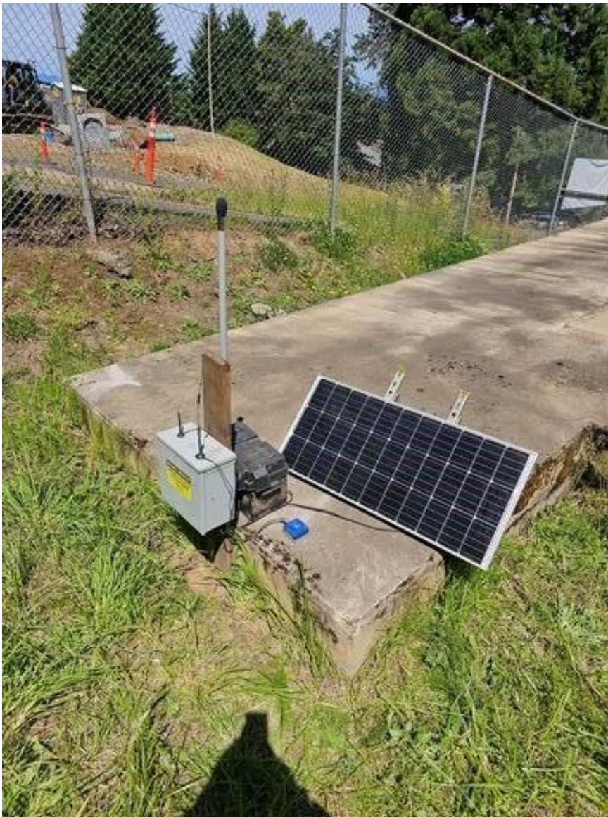
Installed vibration and sound monitors in and around the construction site.
