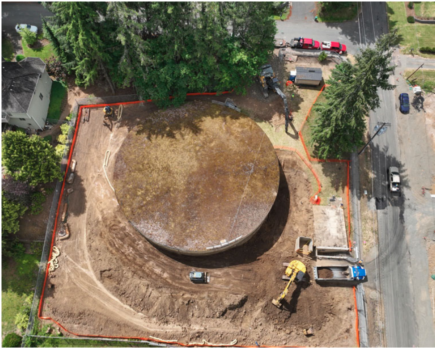
Aerial photo of the 189th Reservoir and Pump Station in July 2024.
