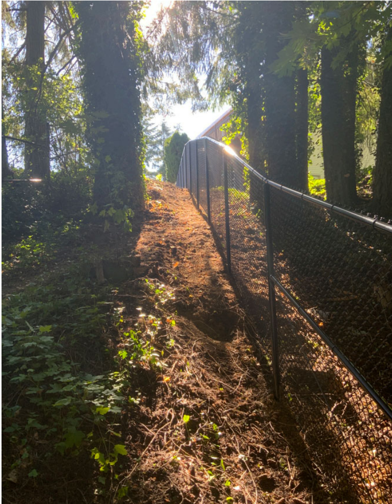
Goyak Reservoir and Pump Station: Photo of the southern fencing
